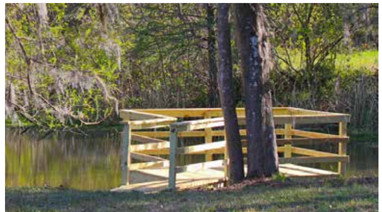
Dock on southern of Oak Lawn removed and rebuilt
