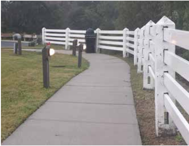
New dock entrance lighting
