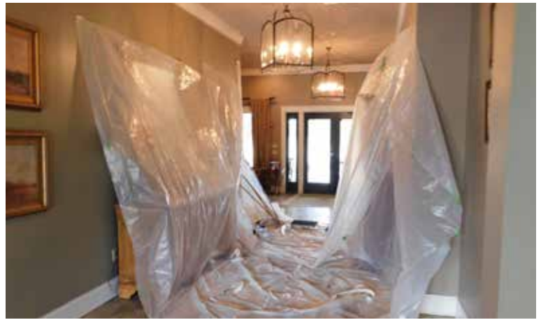
Clubhouse entrance Hallway ceiling repair
